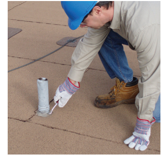
Penetrations require special attention during periodic inspections.
