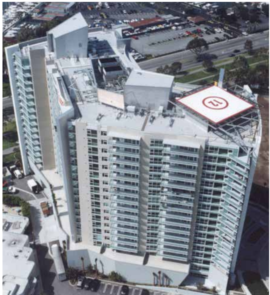
This high-rise luxury condominium tower on the beach at Marina Del Rey, California is protected by a complete Siplast System of torch grade Paradiene and Siplast Lightweight Insulating Concrete.
