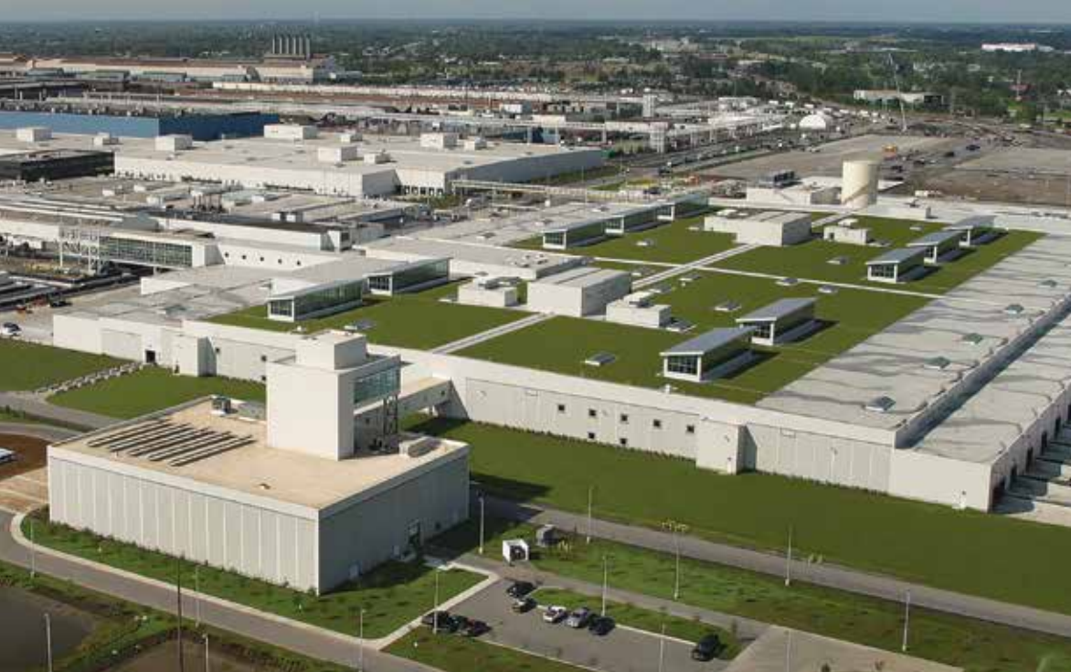
A Siplast Teranap Vegetated Roof System was installed on this automobile manufacturing facility in Michigan, creating the world's largest green roof.
