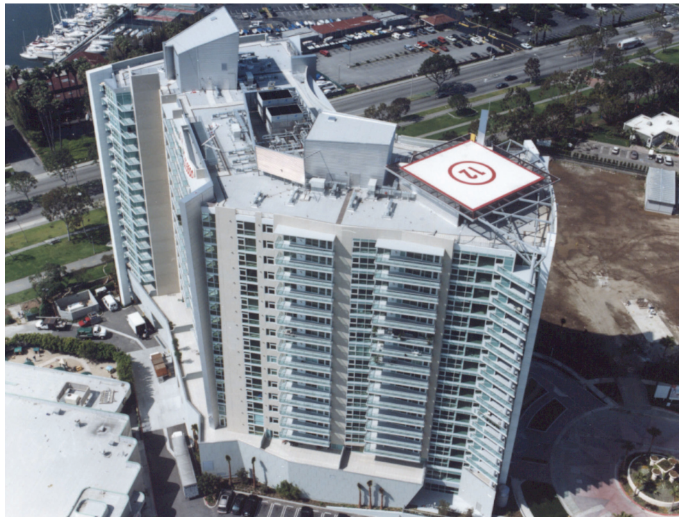
This high-rise luxury condominium tower on the beach at Marina Del Rey, California is protected by a complete Siplast System of torch grade Paradiene and Siplast Lightweight Insulating Concrete.
