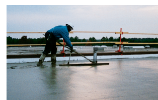
Siplast Lightweight Insulating Concrete is screeded to a smooth, durable, monolithic surface ideal for roofing application.
