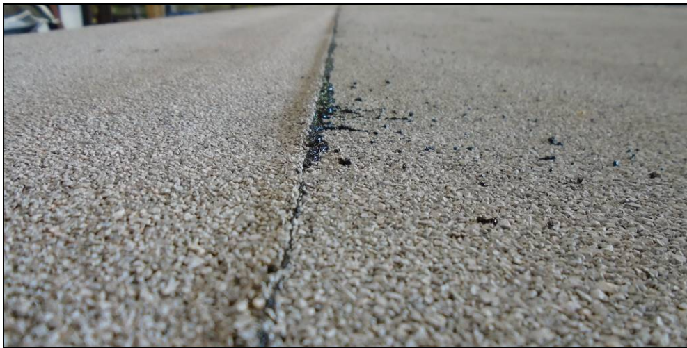
Photo C-10 – Cap sheet overlap joint heat welded
