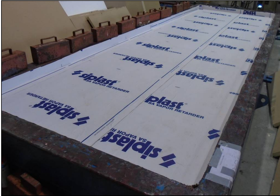
Photo C-3 – Siplast SA Vapor Retarder self-adhered to thermal barrier
