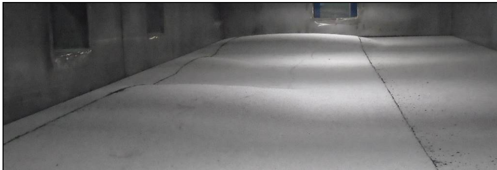
Figure 4 – Blister observed to propagate at different locations
