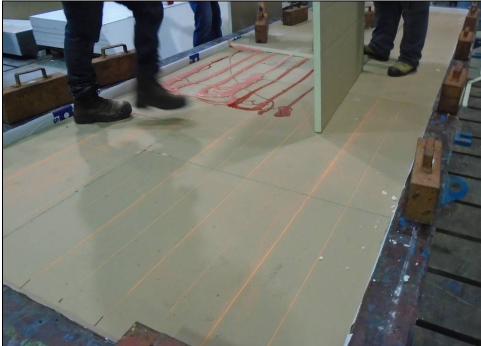
Photo C-5 – Paratherm Insulation (top layer – staggered from bottom layer) ribbon adhered with Parafast Insulation Adhesive C and weights applied on top
